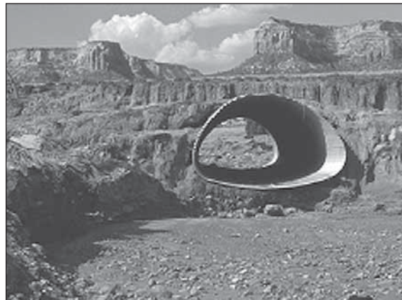
September 7, 1978—South Camp Road culvert exposed. Photo by Jim Johnson.
