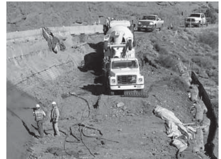
Road construction workers rebuild a collapsed section of Rim Rock Drive.
